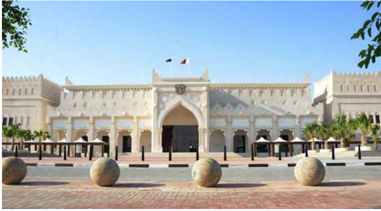
New Traffic & Patrol Department Headquarters [MINISTRY OF INTERIOR (MOI)]
