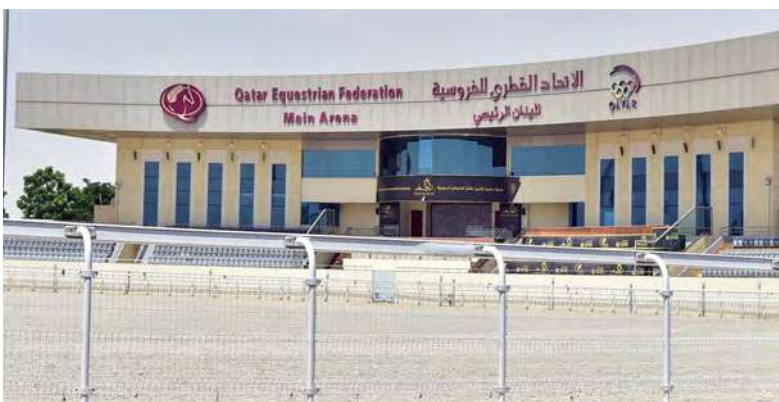
Qatar Racing & Equestrian Federation Facilities [QATAR OLYMPIC COMMITTEE]
