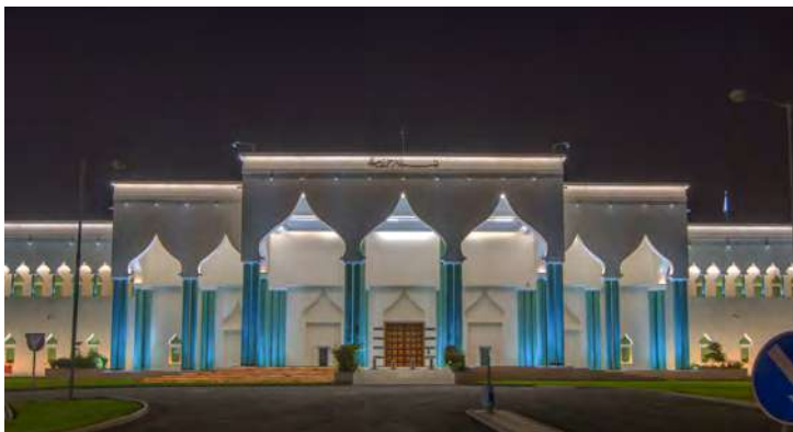
Refurbishment of Amiri Diwan - Phase II [PEO]
